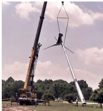
The turbine in hoisted up by a crane.
