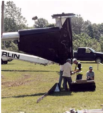
Coxon of SunWind Power and Jolly of Proven, assemble the turbine.
