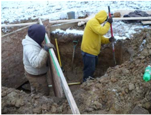
Preparing the foundation for the wind Turbine tower
